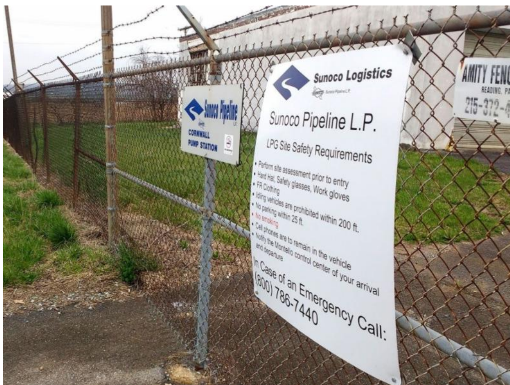
One of the pump stations owned by Sunoco Logistics off of Route 322 near Butler Road in West Cornwall Township.
